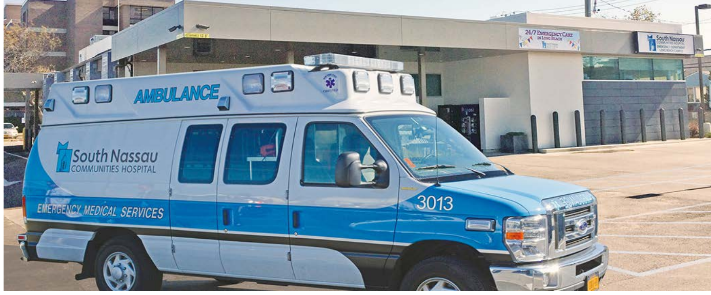
Long Beach Emergency Department
